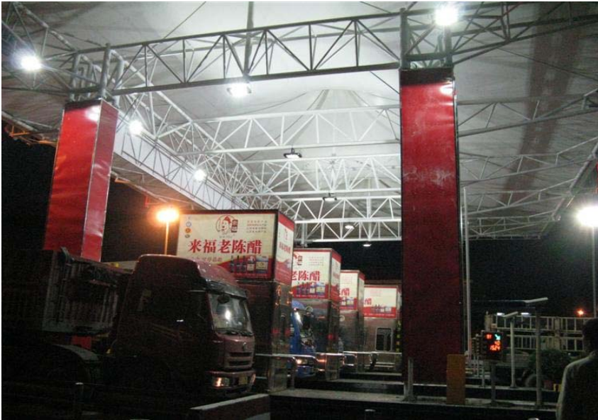
QingXu toll station Illumination Project in ShanXi province
