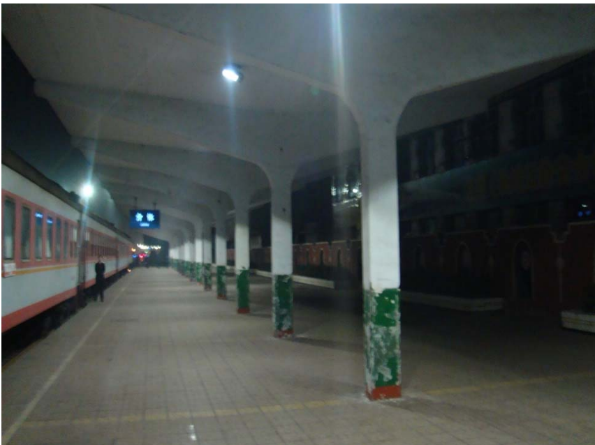
JieXiu railway station platform Illumination Project in ShanXi
