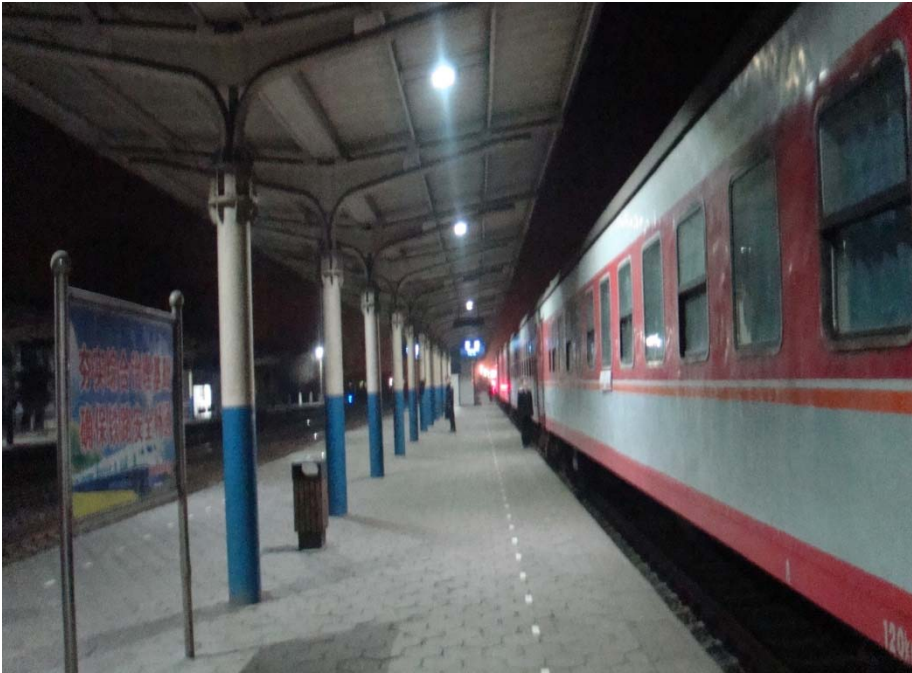
Pin Yao railway station platform Illumination Project in ShanXi
